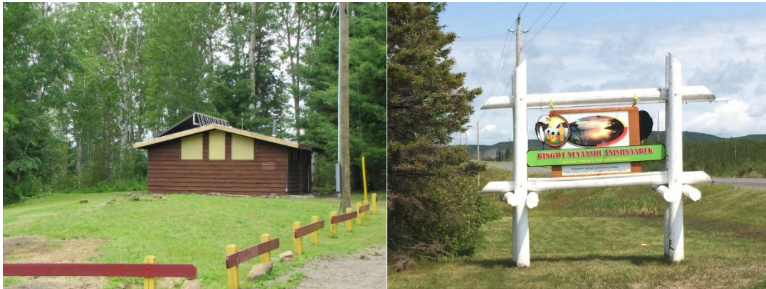
BNA bathroom repaired roof and signage to reserve lands from HWY 11/17
